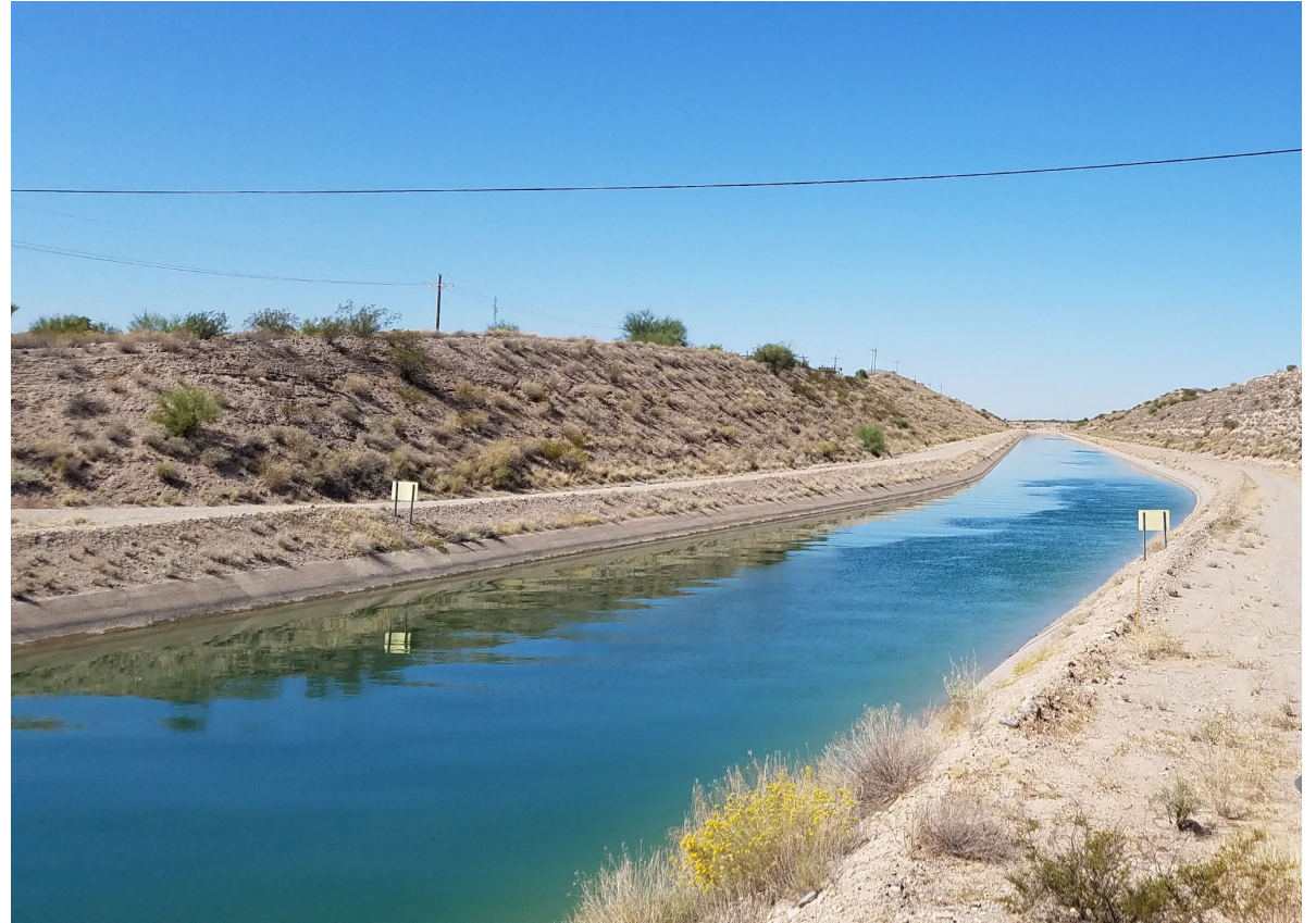
Central Arizona Project Canal near Florence
